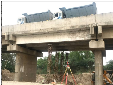
Fig 1: - Bridge Load Testing
