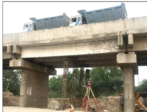
Fig 1: - Bridge Load Testing
