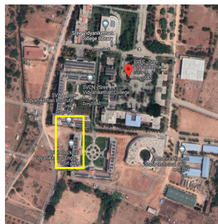
Fig. 1 Building under consideration
