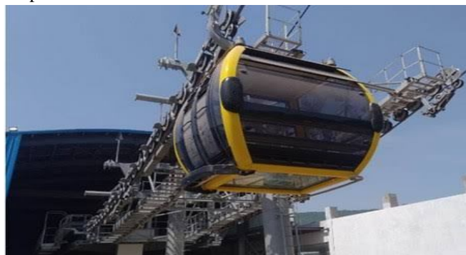
Figure 10: Example of Capsule Ambulance Station at Hospital
