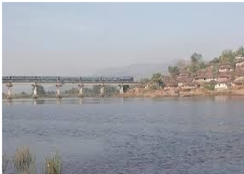
Fig. 5 Railway bridge on Savitri River
