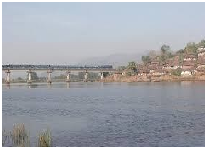
Fig. 5 Railway bridge on Savitri River
