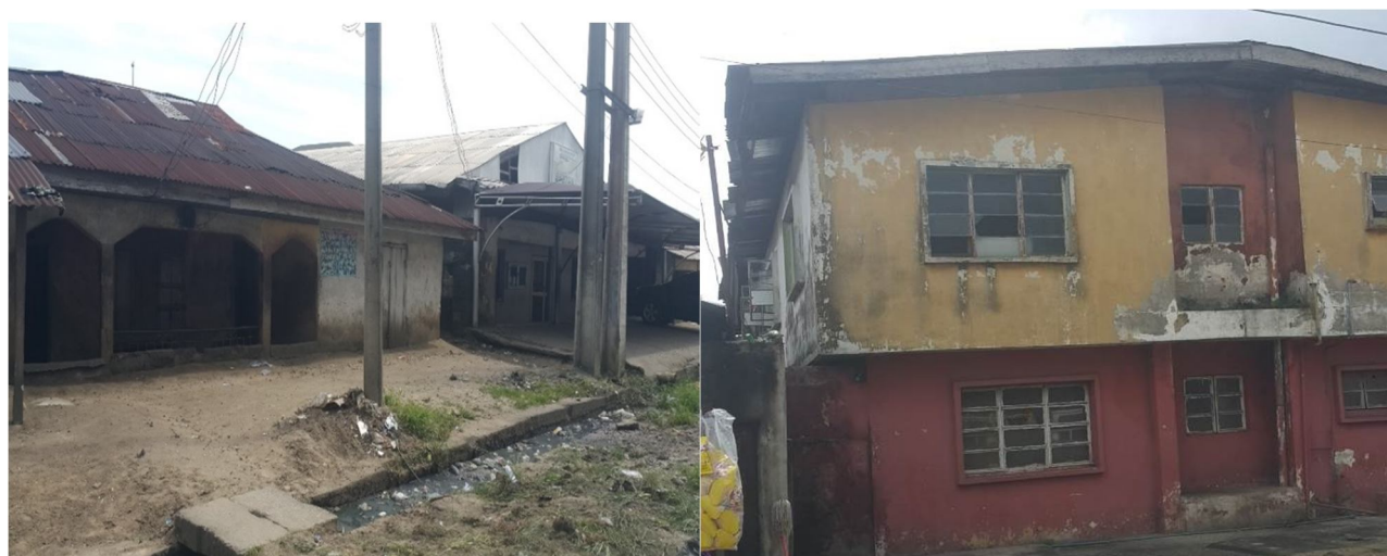
Figure 3: A building in the study area with dampened wall and poor design- floor level is lower than ground level. Figure 4: A building with faded wall paint and broken window glass.
