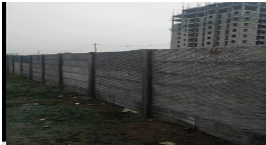
Fig. 8 Precast Compound Walls
