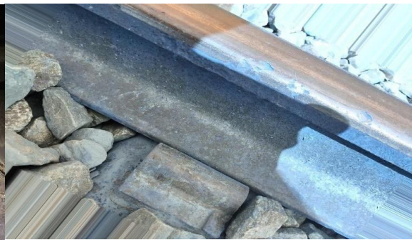
Fig 2 Head checks
