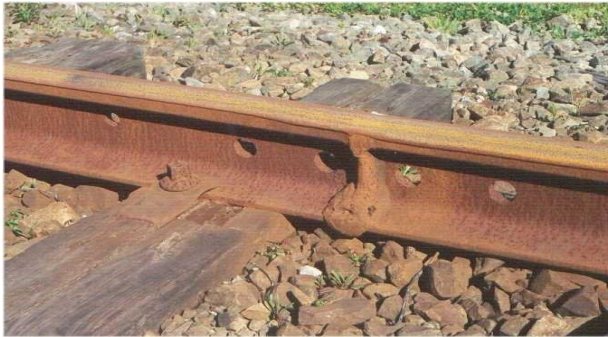
Fig 3 Corrosion
