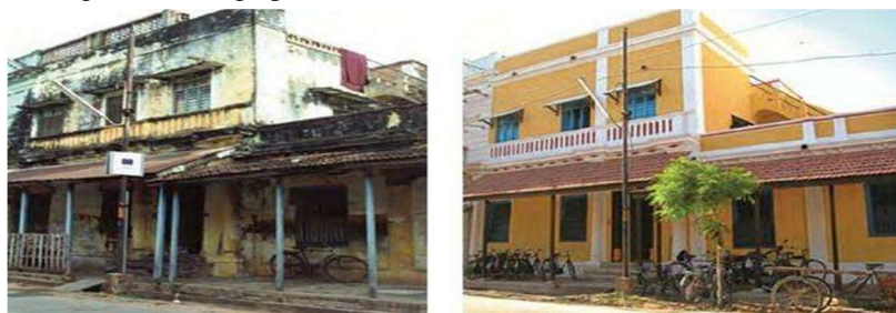
Fig. 3 Houses In Vysial Street Before(left) And After (right) Restoration in Pondicherry (Picture Courtesy: National Institute of Urban Affairs: Compendium Of Good Practices)
