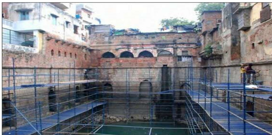
Fig. 1 Hazrat Nizamuddin Baoli renovation (Picture Courtesy: https://www.nizamuddinrenewal.org )
