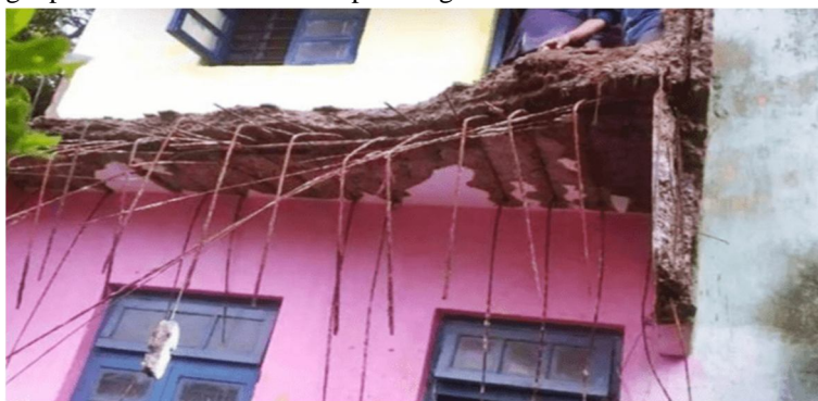
Fig. 8 Balcony of a Rly. quarter collapsed due to heavy rains in Nagpur (Picture Courtesy: https://timesofindia.indiatimes.com/city/nagpur/miraculous-escape-as-rly-quarter-balcony-collapses/articleshow )
