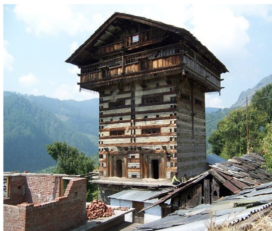
Fig.02 Koti Banal House (Source: https://madhusudanks.wordpress.com/2015/11/07/koti-banal/ )
