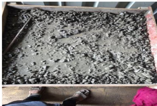
Fig-2: Concreting of conventional slab
