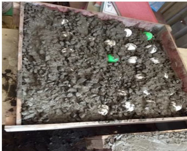
Fig-4: Concreting of Bubble deck flat slab
