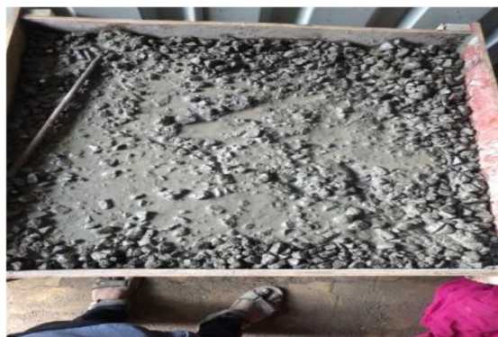
Fig-2: Concreting of conventional slab
