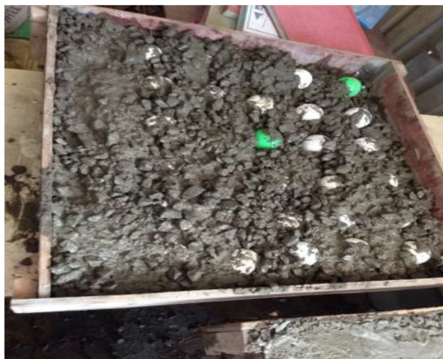
Fig-4: Concreting of Bubble deck flat slab
