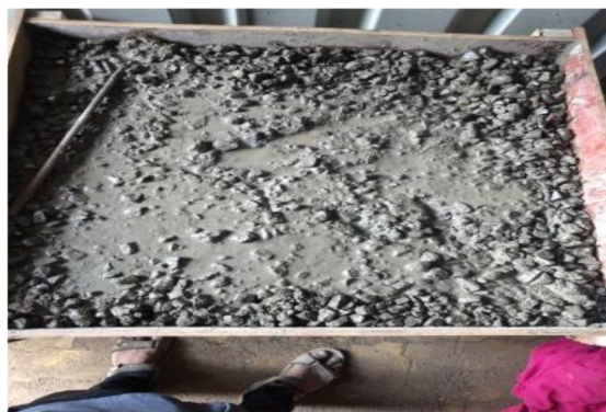
Fig-2: Concreting of conventional slab
