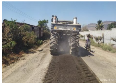
Fig. 2 Mixing with CTSB machine
