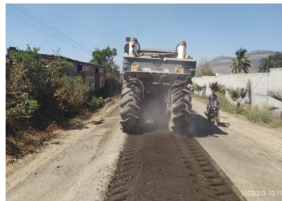
Fig. 2 Mixing with CTSB machine
