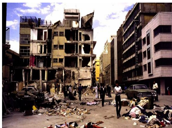
Collapsed buildings with mass irregularity
