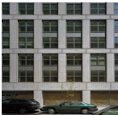
Building with floating column
