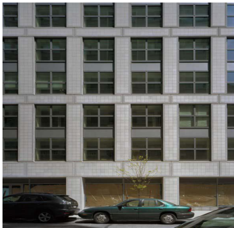
Building with floating column
