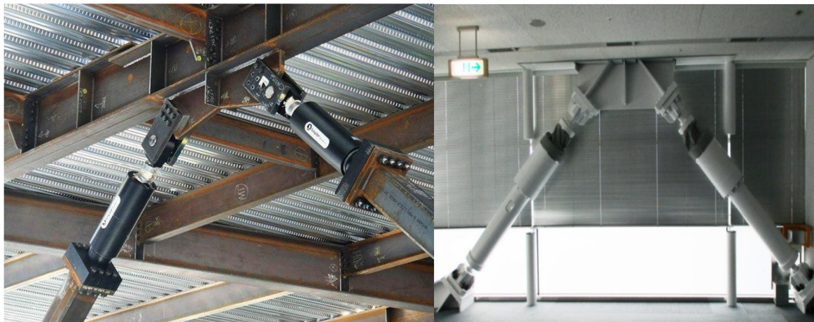
Figure 1.3 Viscous fluid damper
