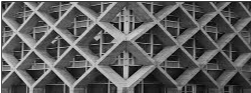
Figure 2: Concrete Diagrid Structural System
