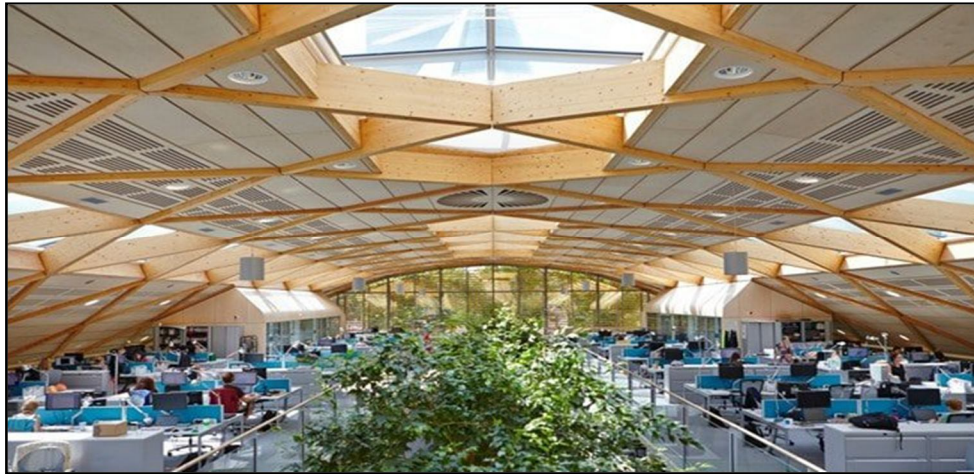
Figure 3: Timber Diagrid Structural System
