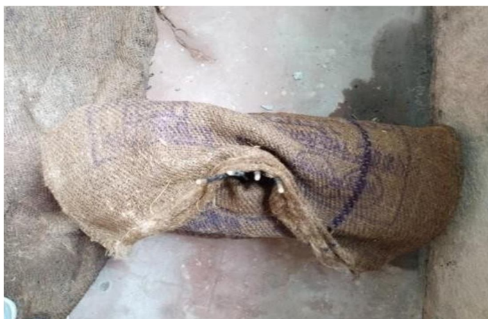
Fig.No.3.17) Curing of Beam
