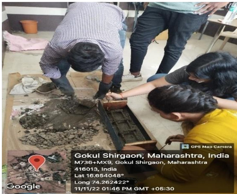
Fig.No.3.14) Casting of concrete
