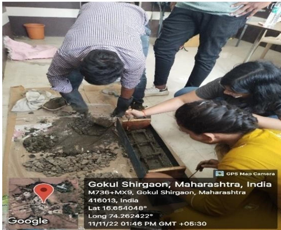
Fig.No.3.14) Casting of concrete
