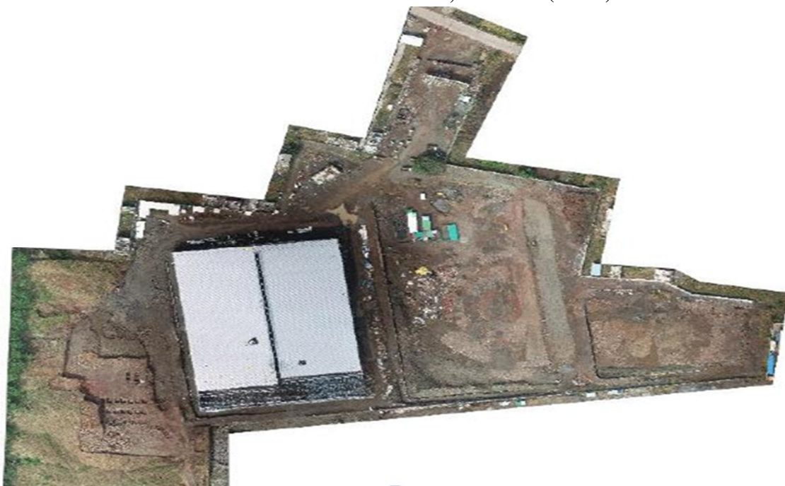
Figure 10: Malpani logistic park, Pune.
