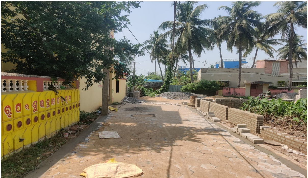
Figure 2.1: Filling The Gaps in between the blocks using sand
