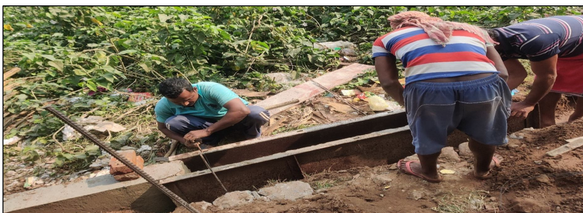
Figure 1.6: Construction of Guard Wall
