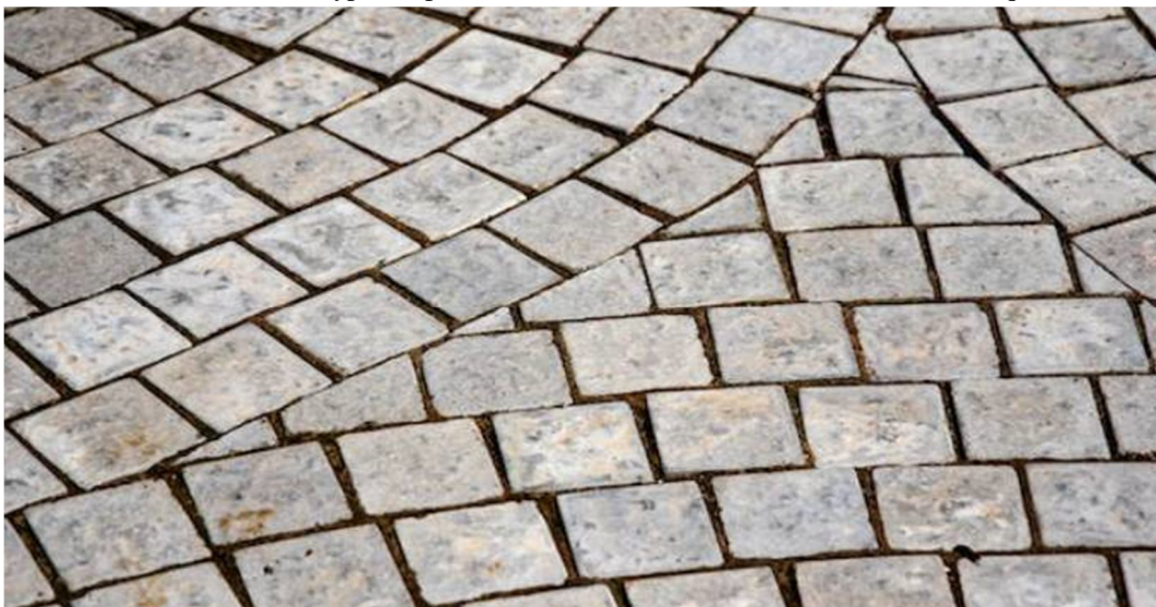
Figure 1.1: Picture Showing Paver Pavement
