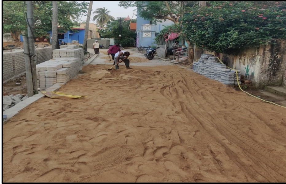
Figure 1.7: Sand Filling Process
