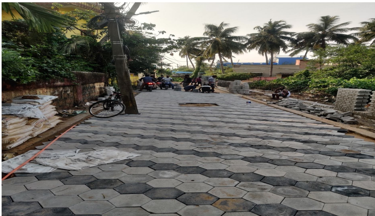
Figure 2.0: Final Cement Concrete Pavement Using Paver Blocks
