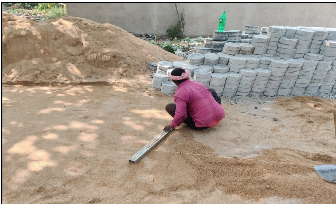
Figure 1.8: Bedding and Sand Levelling
