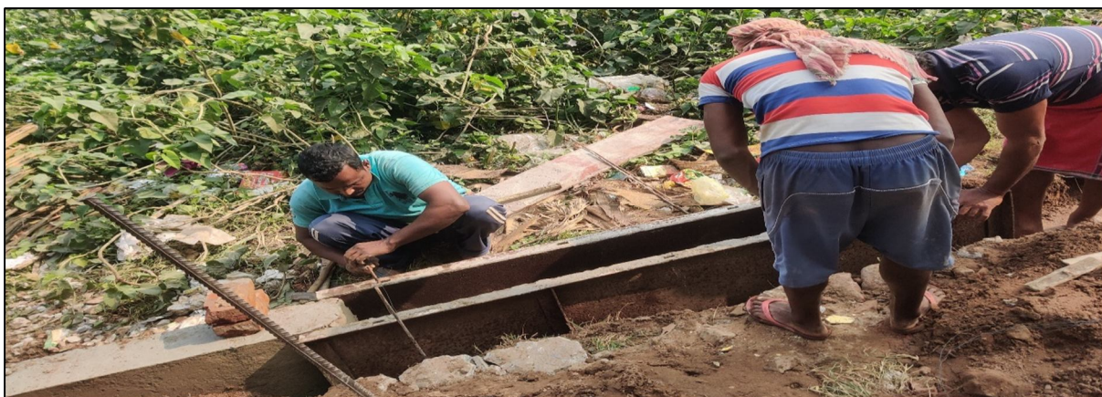
Figure 1.6: Construction of Guard Wall
