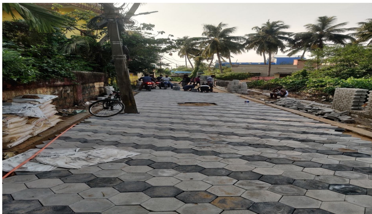
Figure 2.0: Final Cement Concrete Pavement Using Paver Blocks
