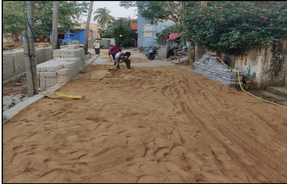
Figure 1.7: Sand Filling Process
