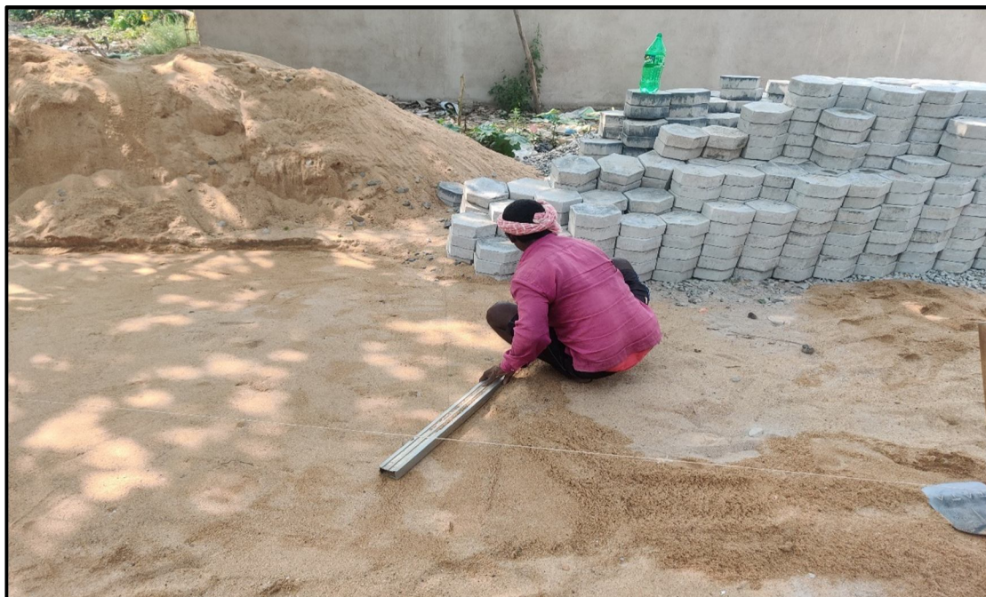
Figure 1.8: Bedding and Sand Levelling
