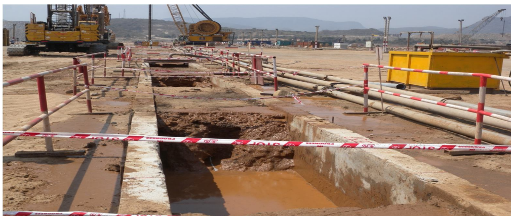
Fig 10. Excavation of primary panel elements
