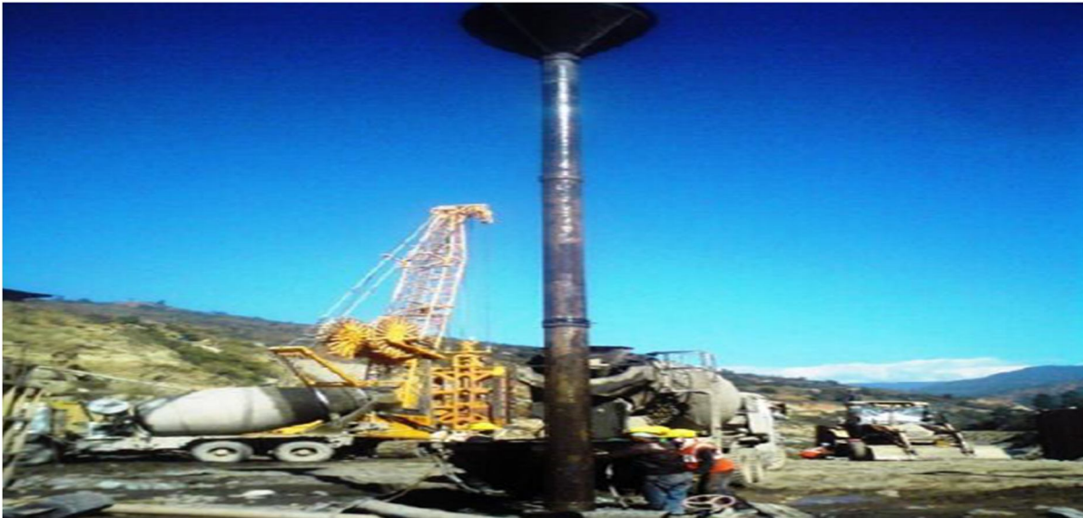
Fig 11.1. Concreting of Panels via Tremie
