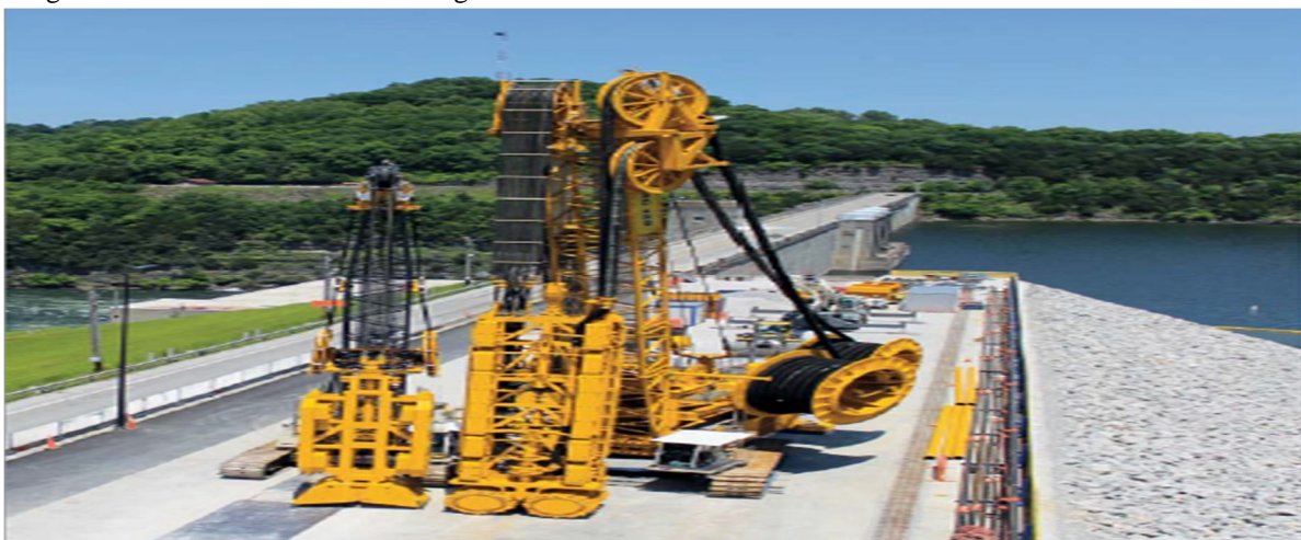
Fig 4. Hydraulic grab and trench cutter
