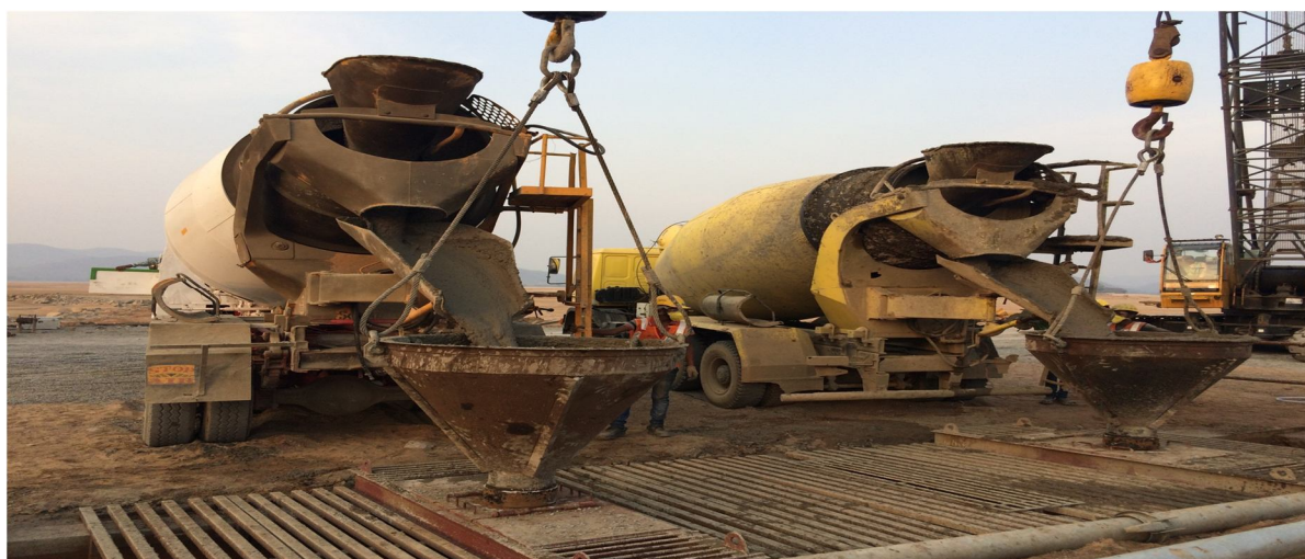
Fig 11.2. Concreting of Panels via Tremie
