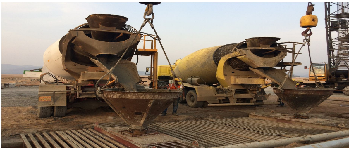
Fig 11.2. Concreting of Panels via Tremie
