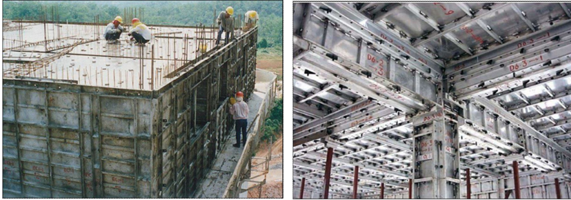
Figure 1.2 Mivan Formwork External and Internal View
