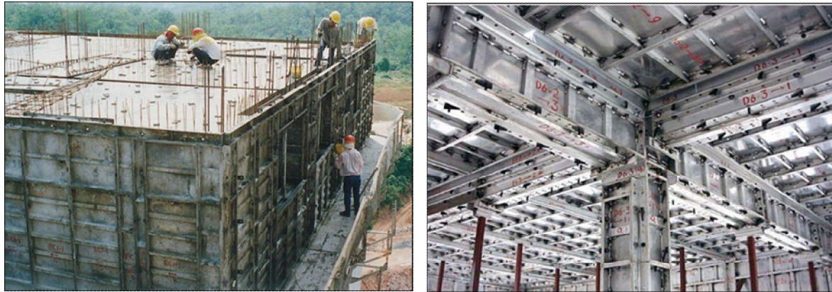
Figure 1.2 Mivan Formwork External and Internal View
