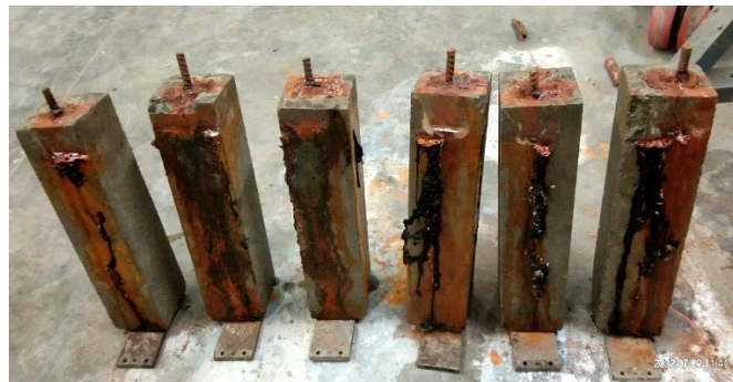
Photograph No. 4.6: Cracks developed due to corrosion on test specimen after 6 cycles.
