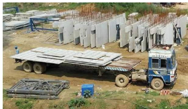
Figure 27: Transport of precast slabs
