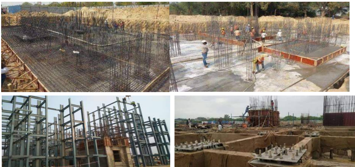
Figure 7: Foundation & Columns in L.H.P.
