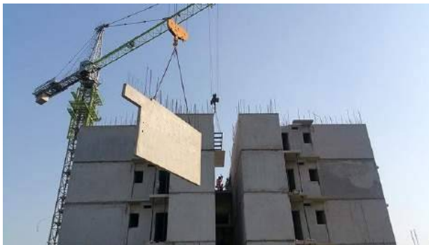
Figure 13: Precast concrete wall erection
