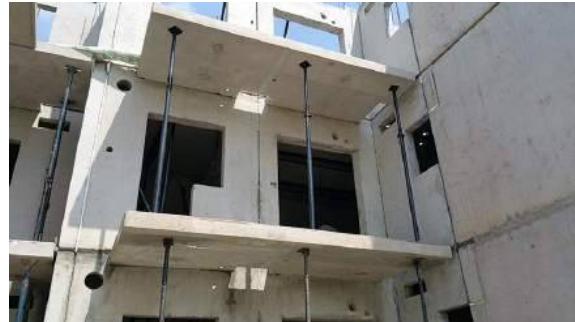
Figure 16: Precast cantilever balconies
