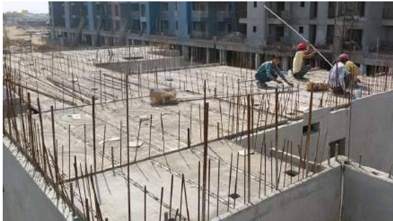
Figure 15: Precast half slab with lattice girder
