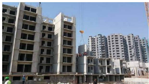
Figure 14: Precast structure on top of basement
