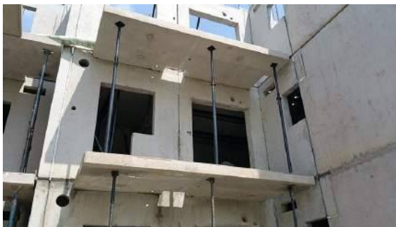
Figure 16: Precast cantilever balconies
