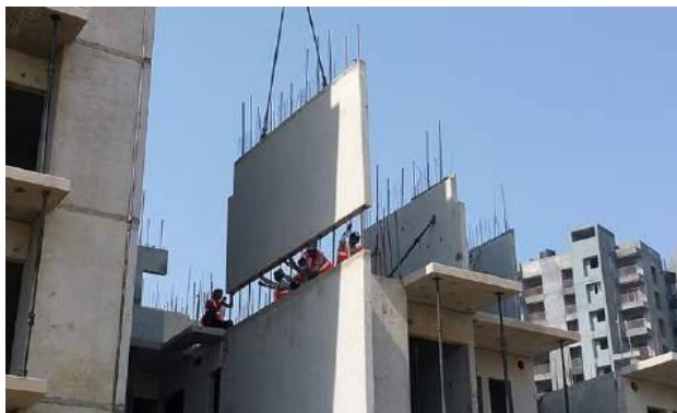
Figure 17: Erection of load bearing Precast wall panel
