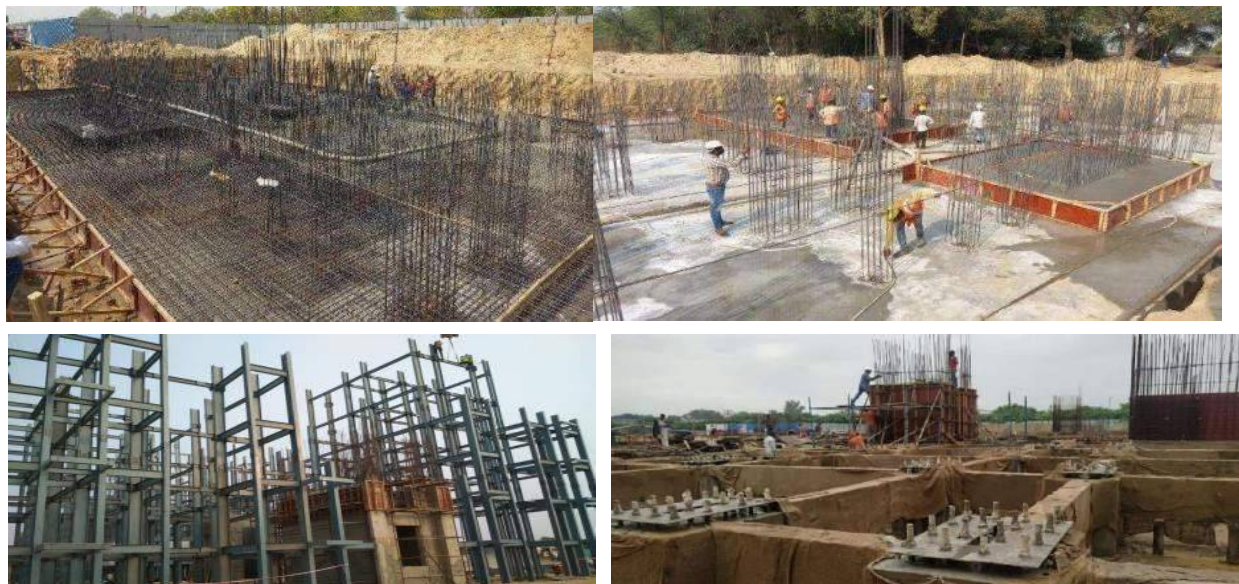
Figure 7: Foundation & Columns in L.H.P.
