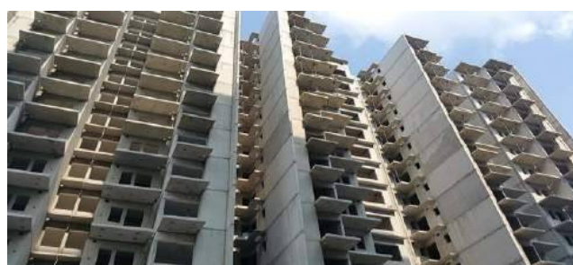
Figure 20: Completed precast building structures
