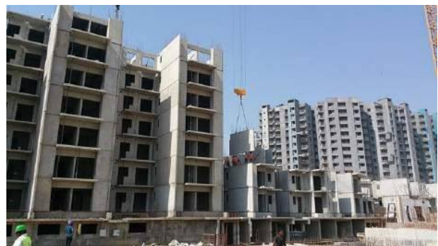
Figure 14: Precast structure on top of basement
