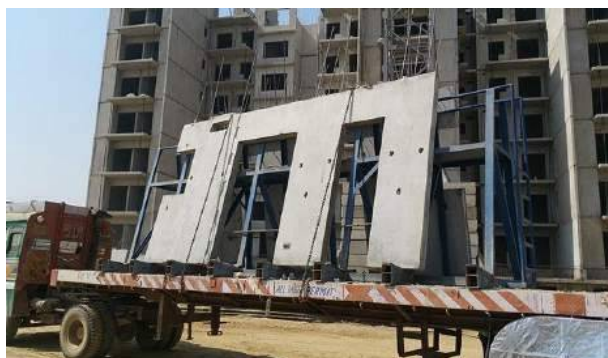
Figure 26: Transport of precast wall panels
