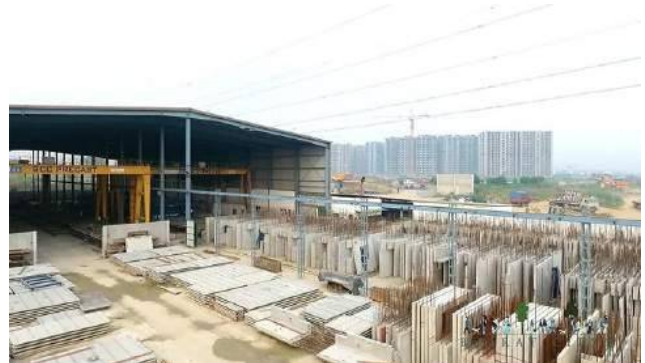
Figure 25: Stockyard for precast elements
