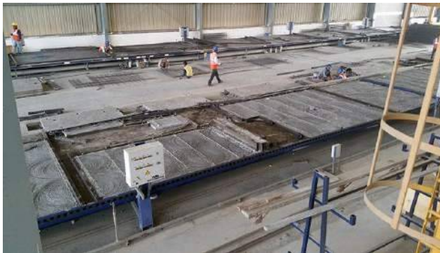
Figure 24: Steel casting beds for Precast slab
