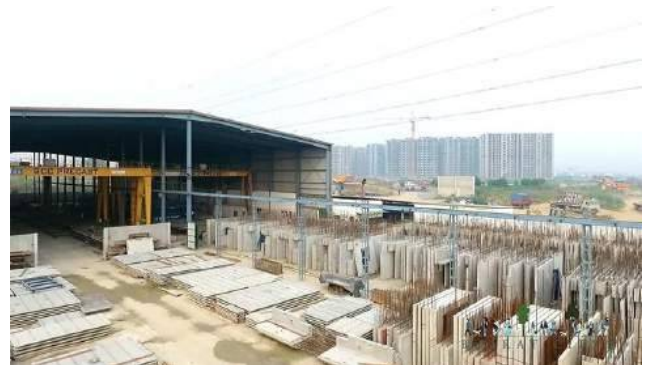
Figure 25: Stockyard for precast elements
