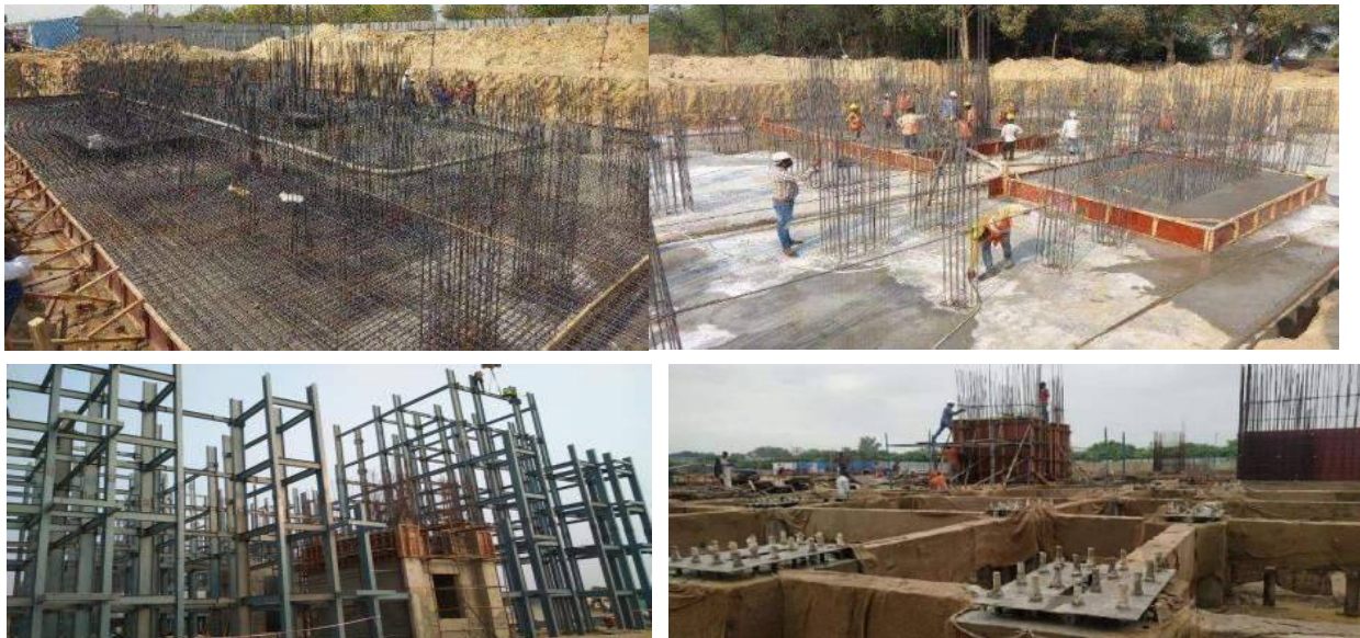
Figure 7: Foundation & Columns in L.H.P.
