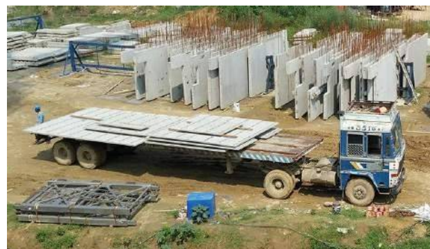
Figure 27: Transport of precast slabs
