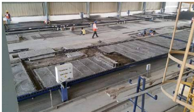
Figure 24: Steel casting beds for Precast slab
