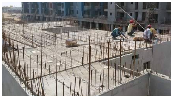
Figure 15: Precast half slab with lattice girder
