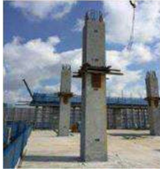
Figure3: Typical Precast Column Details
