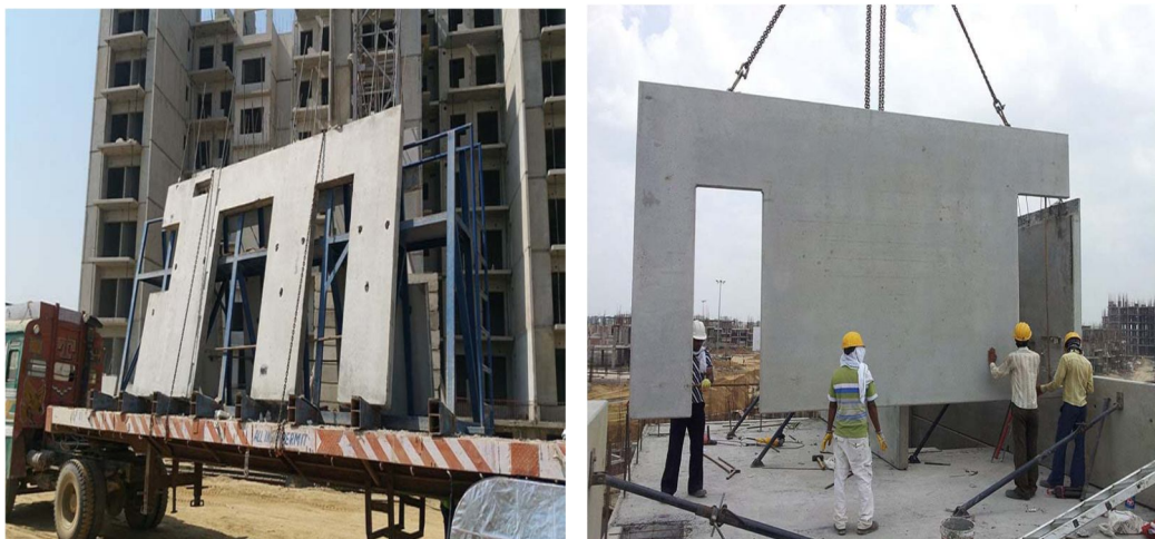
Figure5: Precast wall panels
