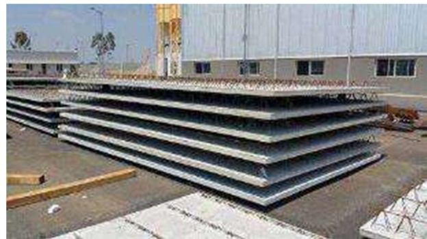
Figure 2: Precast half Slab
