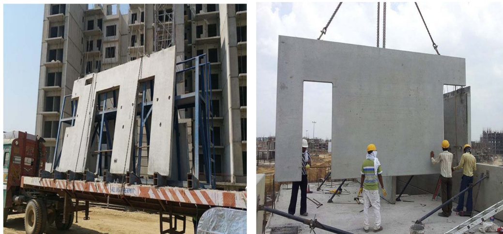
Figure5: Precast wall panels
