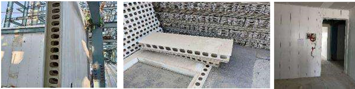
Figure7: PVC Wall panels
