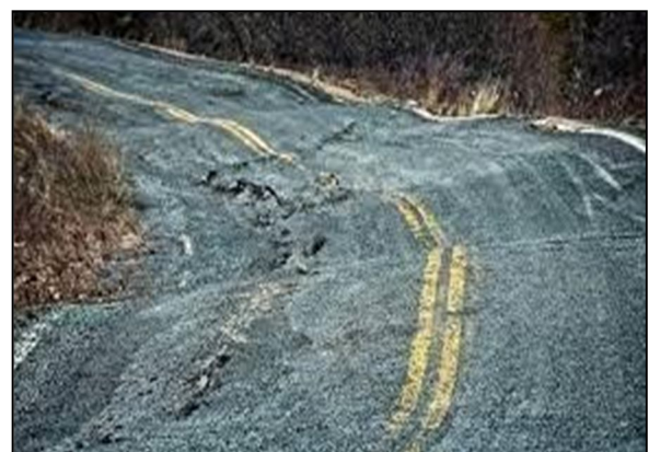
Fig 3.3: Crumbling infrastructure due to thawing of permafrost
