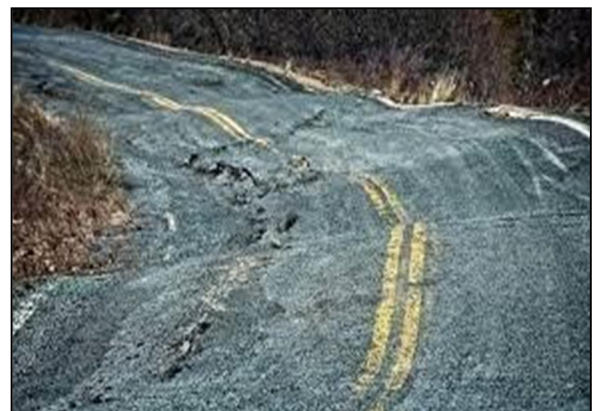
Fig 3.3: Crumbling infrastructure due to thawing of permafrost
