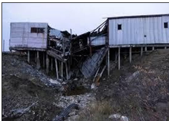
Fig 3.3: Crumbling infrastructure due to thawing of permafrost
