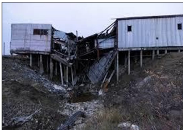
Fig 3.3: Crumbling infrastructure due to thawing of permafrost
