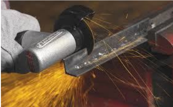
Figure: 35 Metal Cutting
