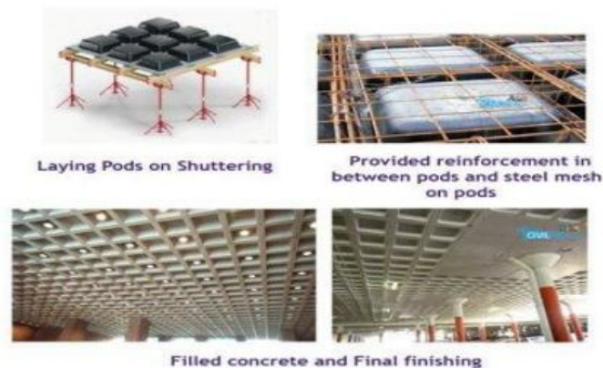
Figure 3: Waffle slab
