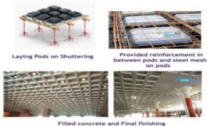
Figure 3: Waffle slab
