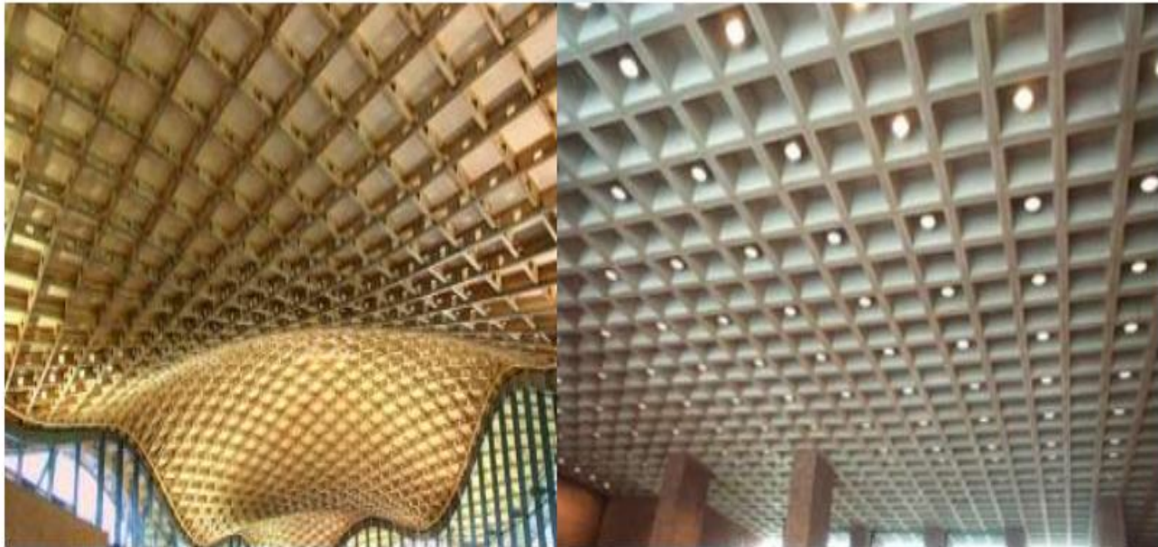
Figure 4: Grid slab
