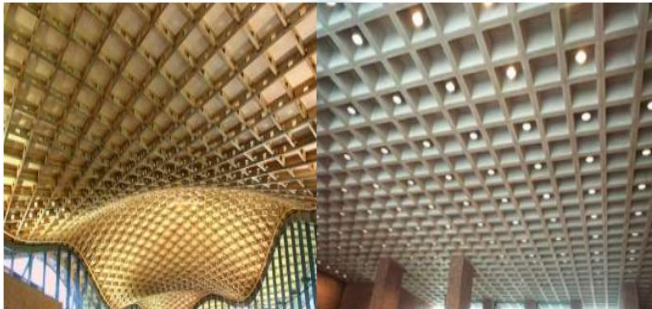
Figure 4: Grid slab
