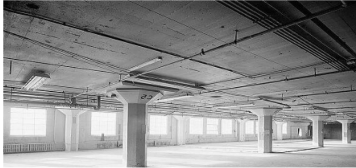
Figure 1: Flat slab
