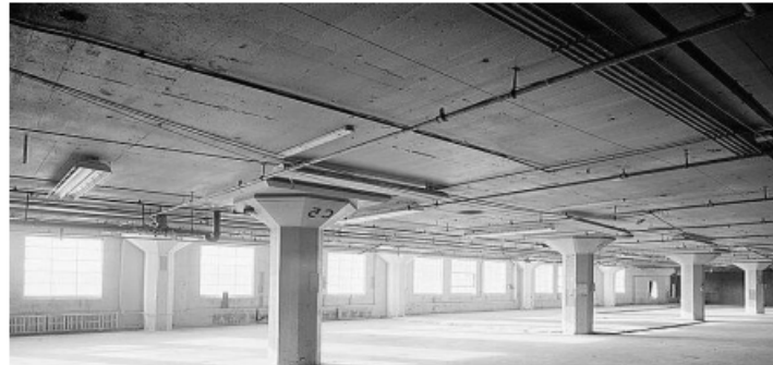
Figure 1: Flat slab
