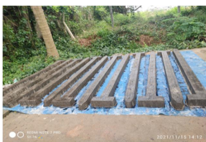
(Fig:- (4)- FINSHING OF FENCING POLE)
