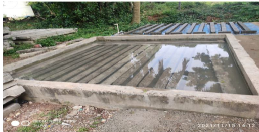
(Fig :- (3)-CASTING & CURING)
