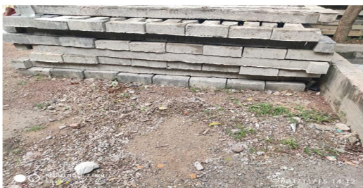
(Fig:- (5)- STORAGE OF THE FENCING POLE AFTER FINISHING CONSTRUCTION WORK )
