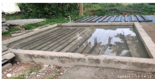
(Fig :- (3)-CASTING & CURING)
