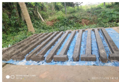
(Fig:- (4)- FINSHING OF FENCING POLE)
