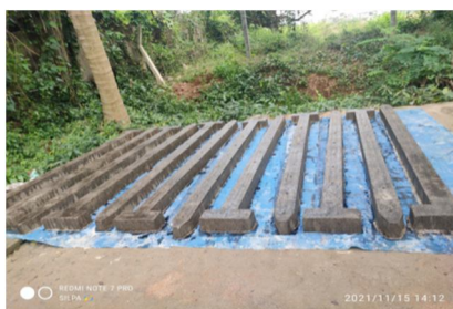
(Fig:- (4)- FINSHING OF FENCING POLE)
