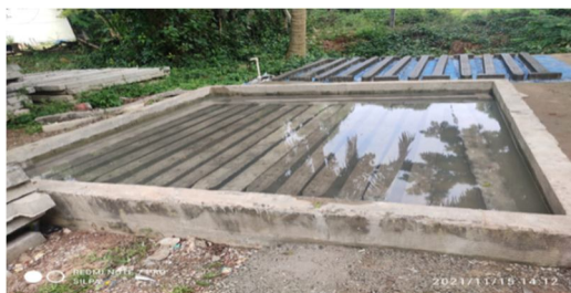
(Fig :- (3)-CASTING & CURING)
