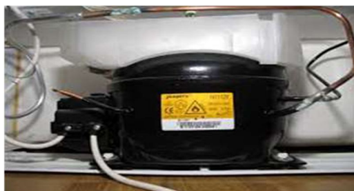
Fig. 2.1: sealed compressor
