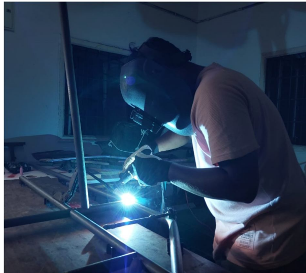
Fig: 7.1.3: Tig welding
