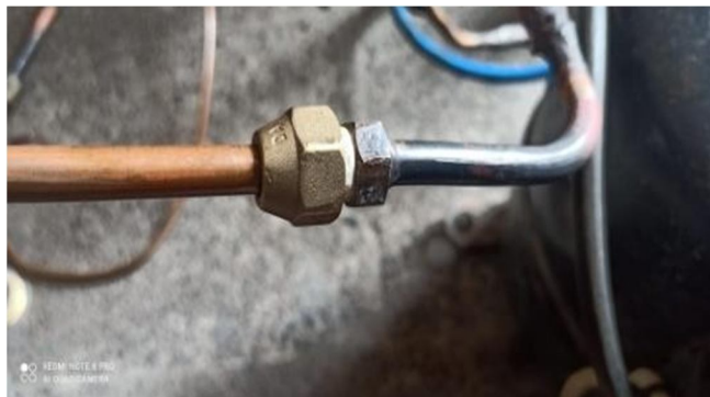
Figure 7: COPPER JOINT
