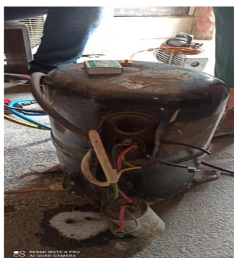
Figure 6: HERMETIC COMPRESSOR
