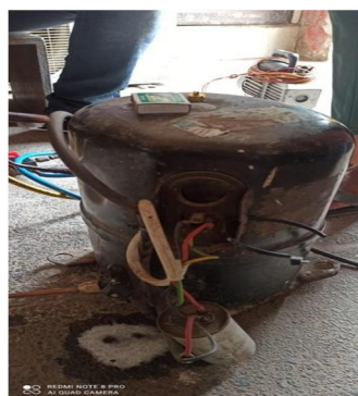
Figure 6: HERMETIC COMPRESSOR
