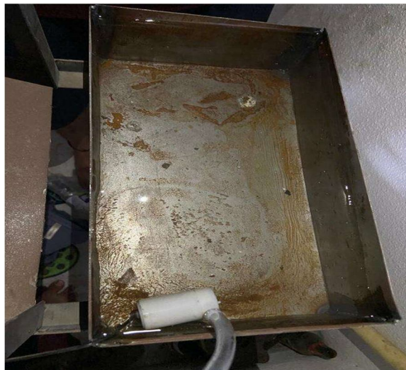
Fig 6 water storage tank
