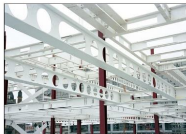
Fig2. Various Opening Shapes In Cellular Floor Beams
