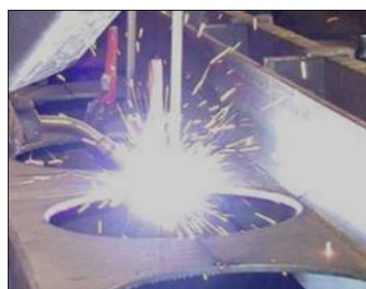
Fig4. Fabrication Process: Welding The Separated Tee-Sections Together
