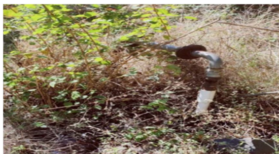
FIG 5. Existing Bore well
