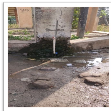
Fig. 3 Condition of existing ESR
