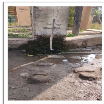
Fig. 3 Condition of existing ESR
