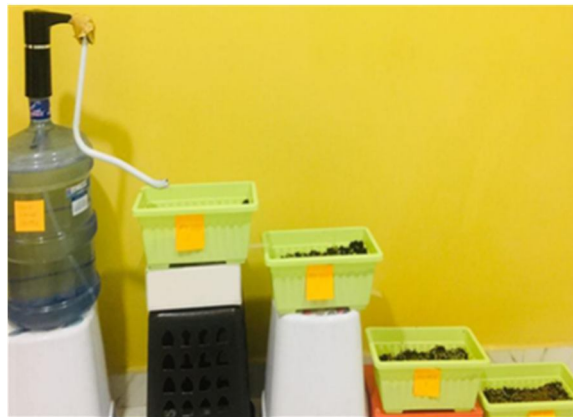
Figure 12: Bio-bed filter setup process in Grey Water Treatment Plant.
