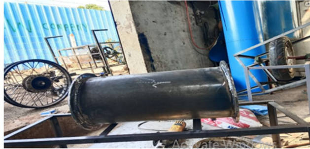
Figure 28 Fabrication of Shell
