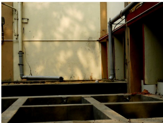
Rain Water Harvest System & Fish Tank
