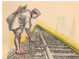
Figure 3. Manual crack detection by human
