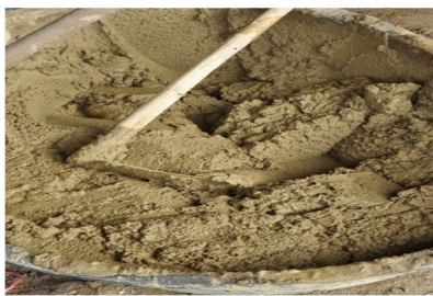
Fig. Soil mixing
