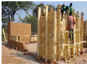
fig. Formwork
