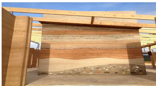
Fig. Developed Rammed earth wall panel
