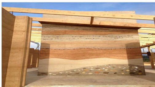
Fig. Developed Rammed earth wall panel
