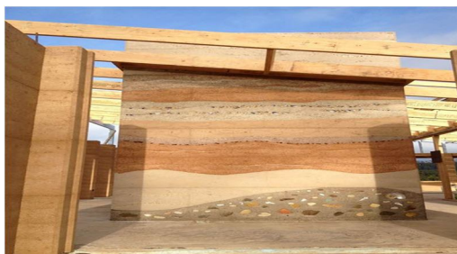
Fig. Developed Rammed earth wall panel
