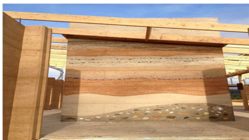
Fig. Developed Rammed earth wall panel
