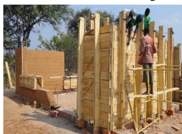
fig. Formwork
