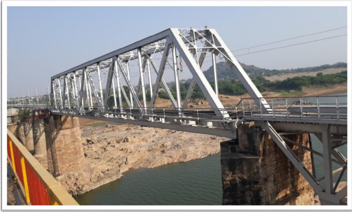
Fig. 1 : Existing Railway Steel Bridge (Ken Bridge) at City Banda
