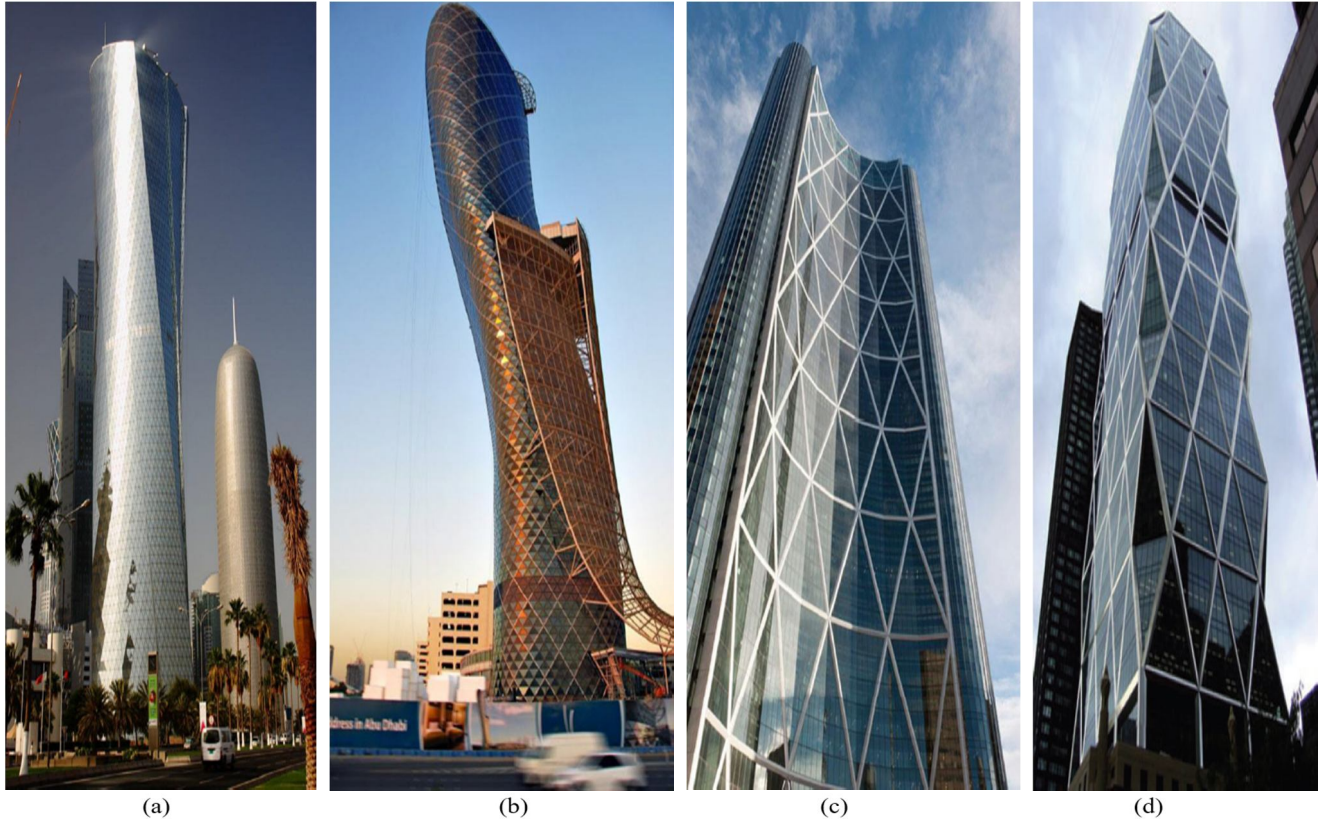
Fig.1 (a) The 44-story Al Bidda Tower in Doha, Qatar (b) The Capital Gate, Abu Dhabi (c) The Bow tower, Calgary, Canada (d) Hearst Headquarters, New York
