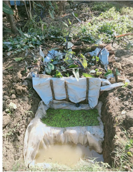
Fig. 9: Completed Reed bed filter with Colocasia esculenta and Pistia stratiotes / Spirodela and lamna
