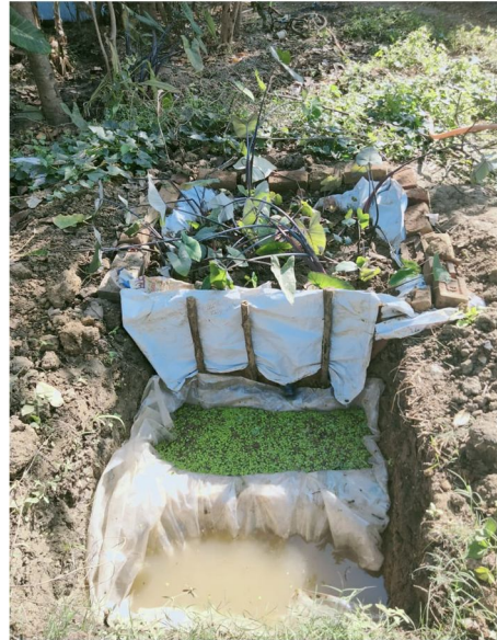
Fig. 9: Completed Reed bed filter with Colocasia esculenta and Pistia stratiotes / Spirodela and lamna
