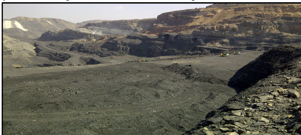
Fig 1 – Typical Coal Mine Road Condition
