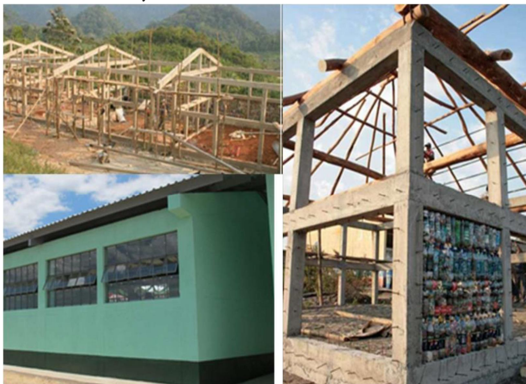
Figure 3-1 Construction process of a bottle school built by Hug It Forward in Guatemala 1) Completed school, plastered and painted (2019)
