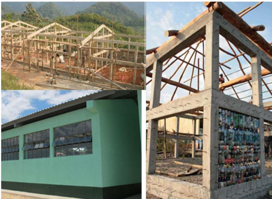
Figure 3-1 Construction process of a bottle school built by Hug It Forward in Guatemala 1) Completed school, plastered and painted (2019)
