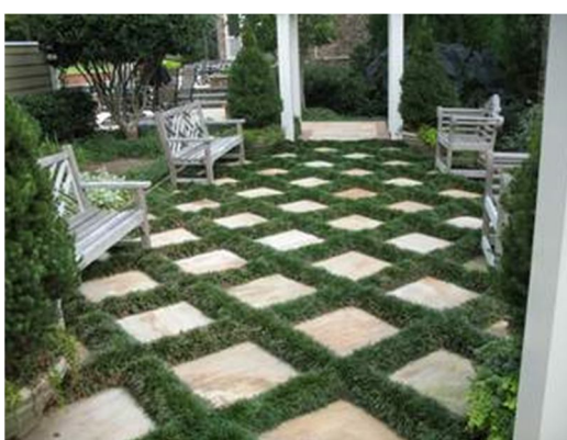
Fig.5 concrete grass pavers with lawn view
