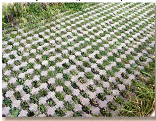
Fig.4 concrete grass pavers
