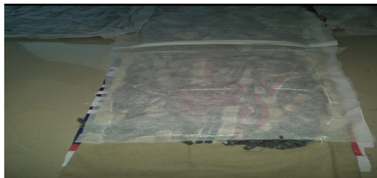
Fig 4. Efficient curing pad for curing to concrete
