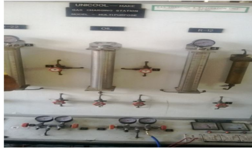
Fig.9:- Installation of Refrigerant in Compressor
