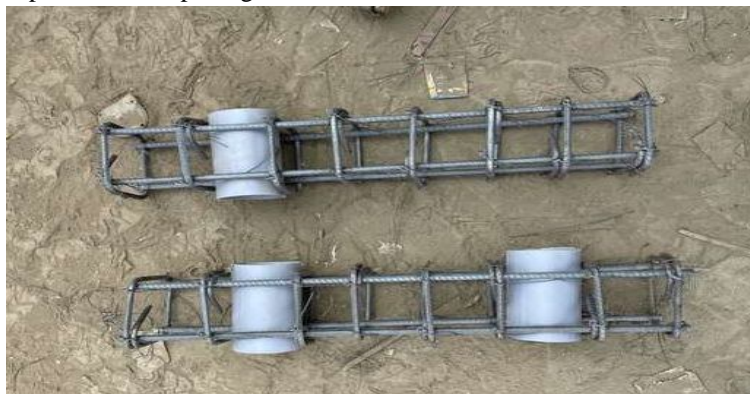
Fig 4.4.1 Reinforcement & Openings
