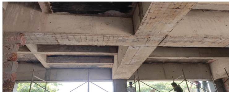
Fig. 3 Primary and Secondary beams in First Floor
