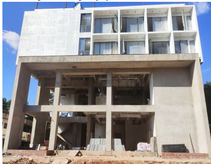
Fig. 1 Front view of Hotel Kaashi Building
