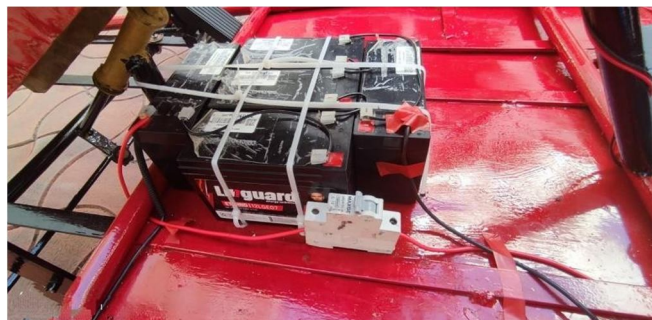
Fig 5. Battery and MCB installation
