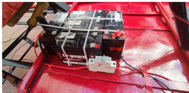
Fig 5. Battery and MCB installation
