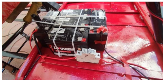
Fig 5. Battery and MCB installation
