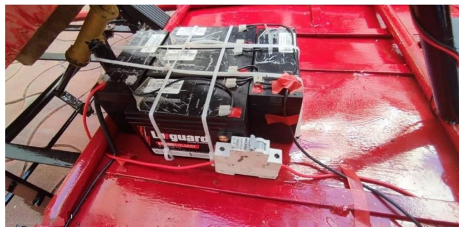
Fig 5. Battery and MCB installation
