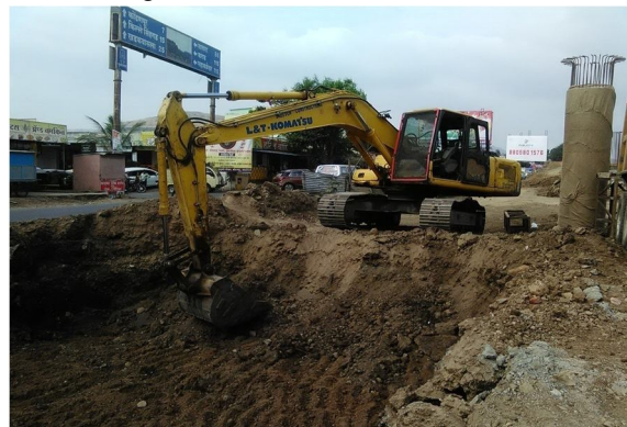
1.3 Excavator (L& T- Komatsu PC-200)
