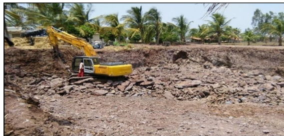
1.2 Excavation by Crawler type excavator-(HYU 220 LC-7)
