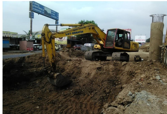
1.3 Excavator (L& T- Komatsu PC-200)
