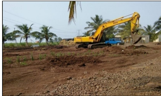
1.1 Excavation by Crawler type excavator-(HYU 220 LC-7)
