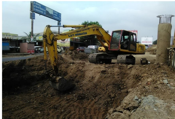
1.3 Excavator (L& T- Komatsu PC-200)
