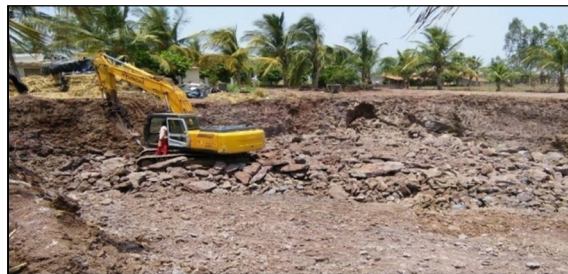
1.2 Excavation by Crawler type excavator-(HYU 220 LC-7)
