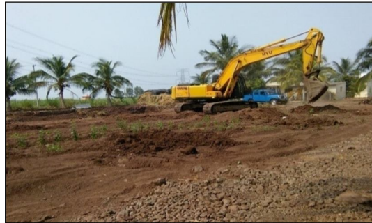
1.1 Excavation by Crawler type excavator-(HYU 220 LC-7)
